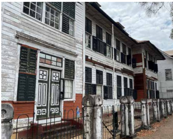
Potential location for housing development at the Herenstraat
