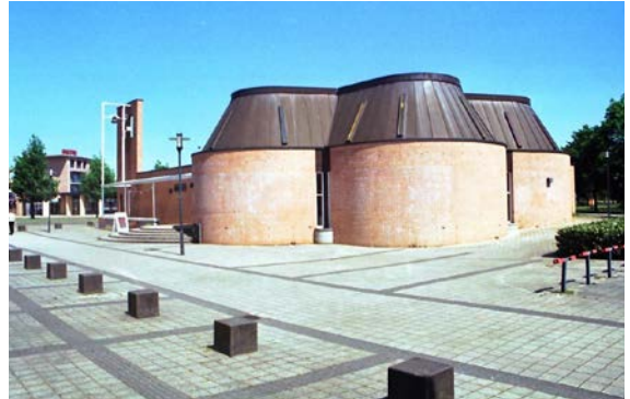
Lucaskerk in Breda, architect H.J. Groeneweg, 1994
