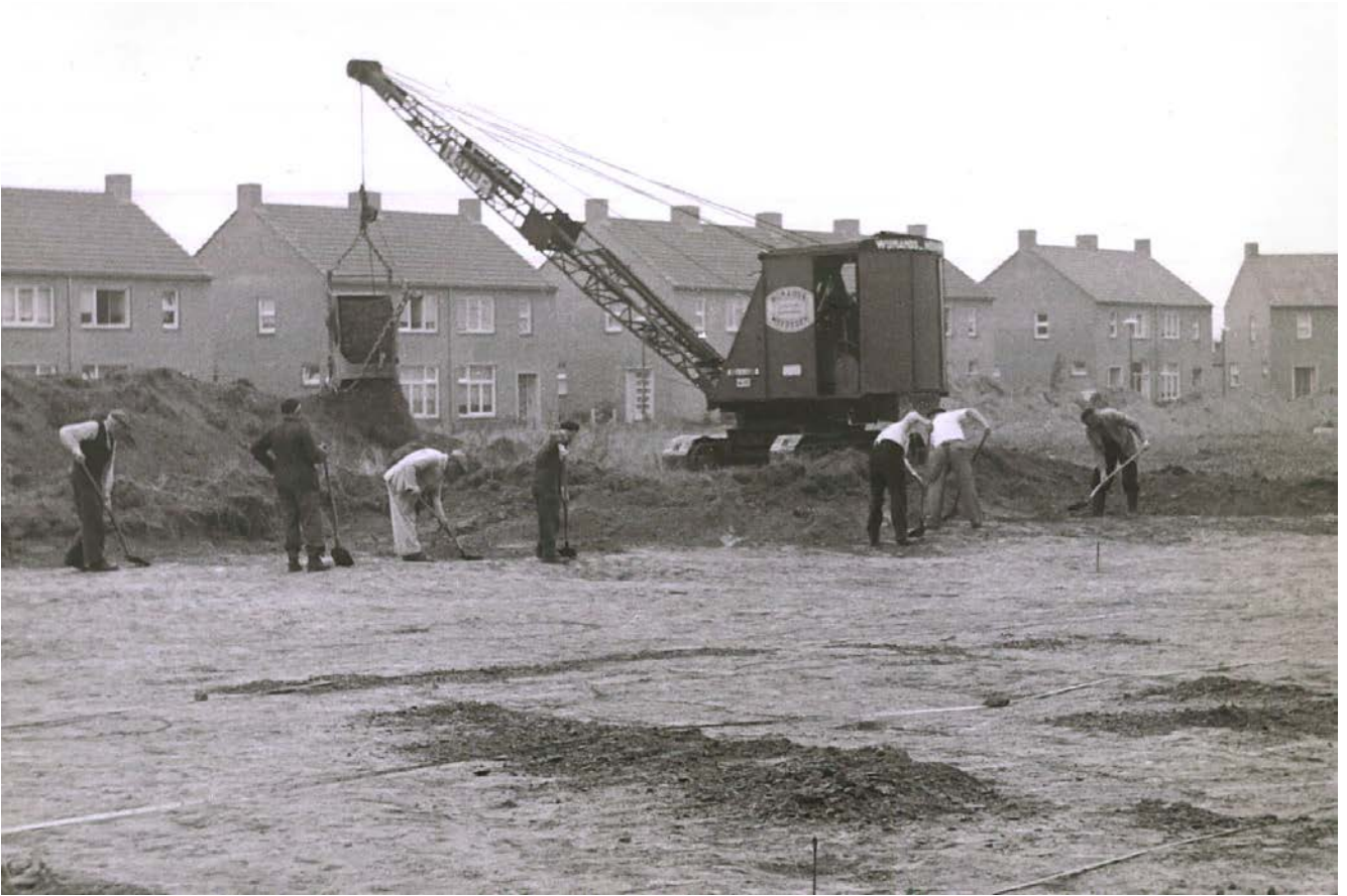
Fig. 6.3 The use of the dragline for removing the topsoil.
