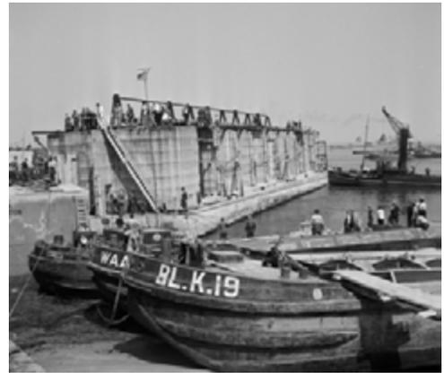
220 The closing of the Braakman tidal inlet by using Phoenix caissons. This pre-1953 operation was one of the hasardous pilot-projects before the North Sea flood struck the south-west. (Photo 1952)
