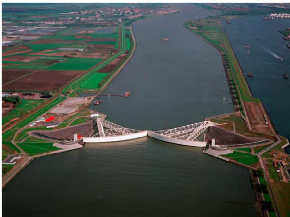
218 Aerial impression of the 1997 Maeslant barrier in the Nieuwe Waterweg - waterway to Rotterdam. Both swinging barrier arms are about 240m. (Photo July, 2007)
