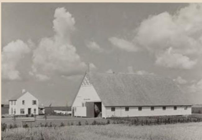
184 Noordoost Polder model farm H.D. Louweshoeve on lot nr. M 109. This concrete barn assembled at location out of prefab elements by Schokbeton Ltd. dates from 1949 and is the first of this type. (Photo 1950)
