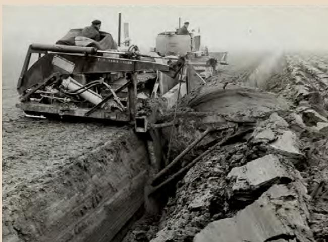
185 Deep ploughing in Noordoost Polder with two 'Caterpillar machines' in line drawing the ploughshares. (Exact place and date unknown).
