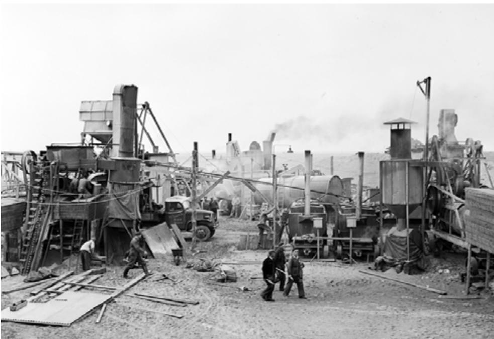
214 Soon after the 1953 disaster dyke repairs claimed the bringing into action of as much as possible of modern equipment. Not only sand, clay and basaltic blocks were used but asphalt-paving was also applied. This picture was taken autumn 1953 near Middelhamnis, island of Goeree-Overflakkee.
