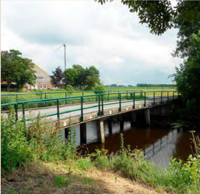
211 Haskerveen Polder. Characteristic bridge in reconstruction period land consolidations etc. Most wooden and stone bridges were replaced by plate girder bridges with deck on concrete piers, as led lack of bridges in punting polders to the building of such specimens. (Photo 2008)
