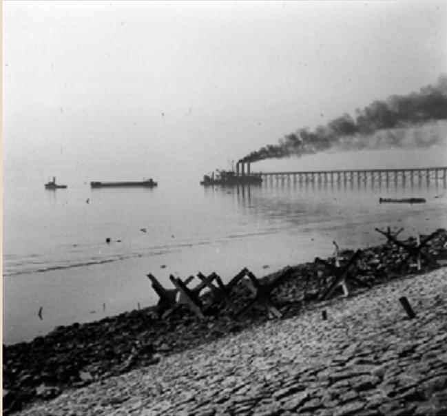
227 Soon after the war the bombed dykes of Walcheren had to be repaired. This picture shows transport of building-materials and a dredger and pipework near Rammekens. Notice the German tetrahedrons that have not yet been removed. (Photo 1946)
