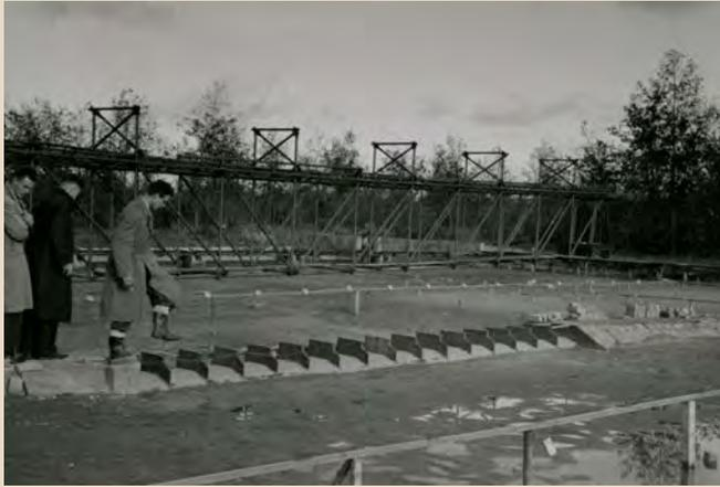
186 This Waterloop Bos (Watercourse Forest) model is a scaled-down experimental water-hydraulic installation for the Haringvliet flood barrier. (Photo probably ca. 1957)
