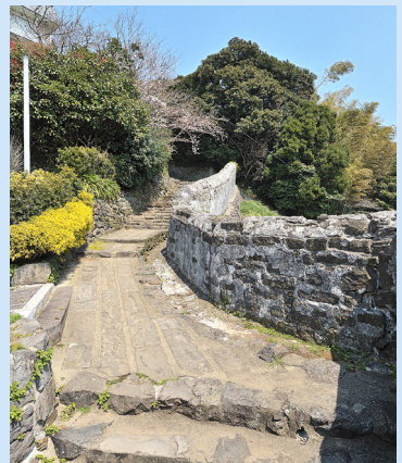
Wall surrounding the VOC-warehouse
