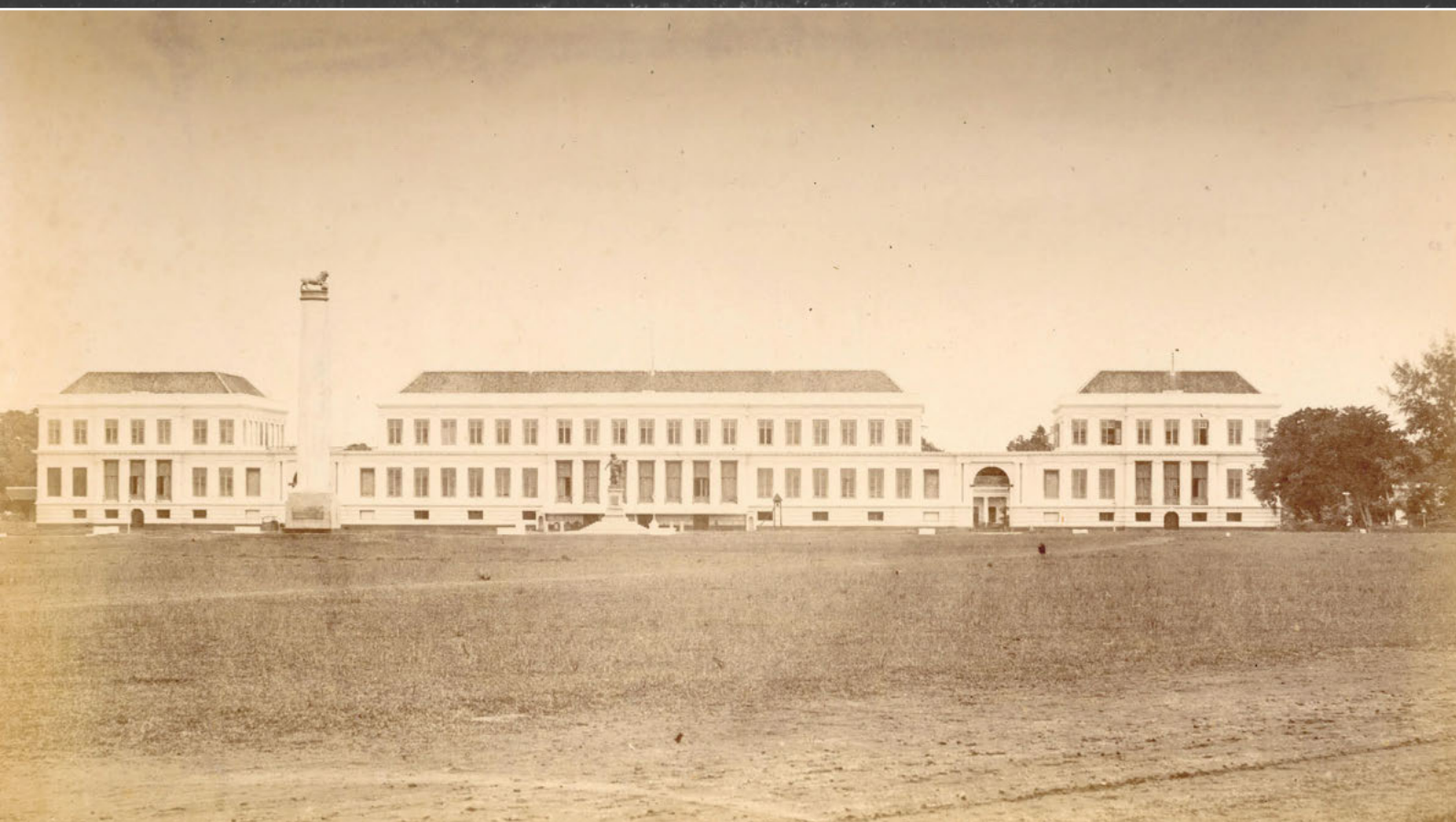
Illustration 6: Photographs (late 19th century) showing the front façade of the Ministry of Finance Heritage Building in Weltevreden, Batavia (now Jakarta).
