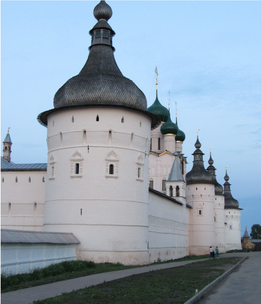
FOTO LINKS: MUREN KREMLIN ROSTOV
