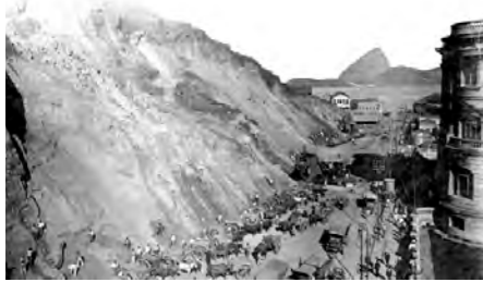
Dismantling of Castle Mountain PHOTOGRAPHY: AUGUSTO MALTA
