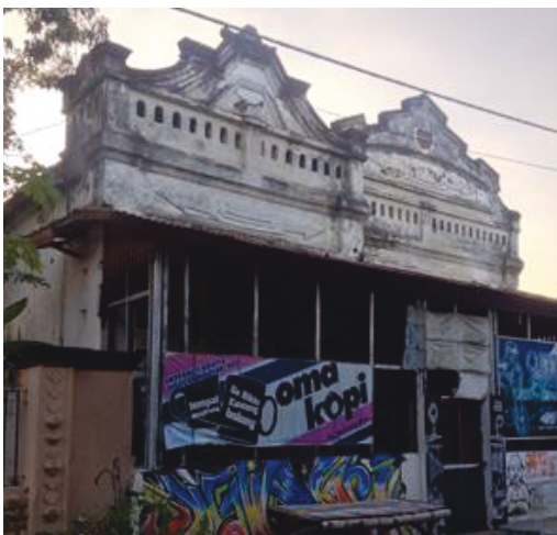
Building in need of maintenance to safe its features (Arab quarter).
