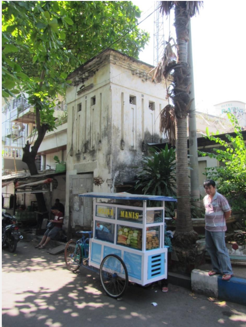
One of the characteristic old electricity buildings.
