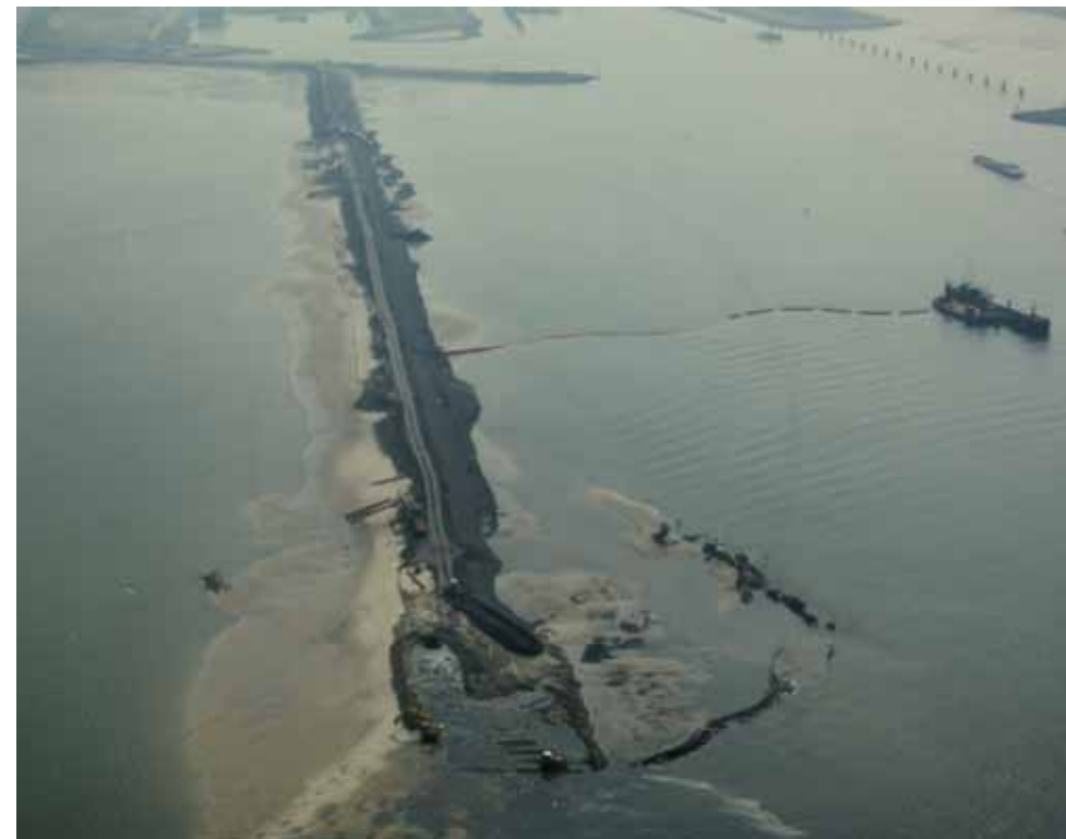
doorgebroken dam [RWS]
