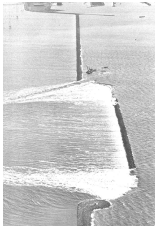
doorgebroken dam [Deltaberichten]
