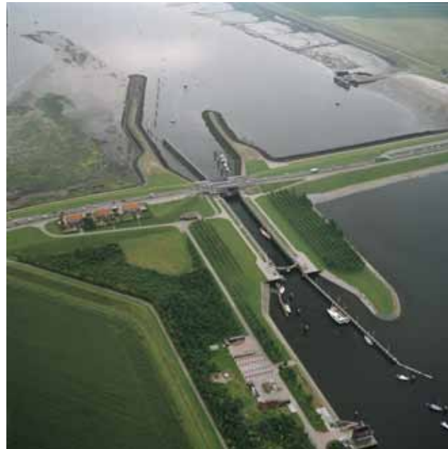
voltooid sluisencomplex [RWS]
