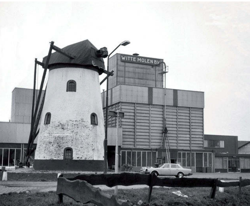
The Witte Molen in Meeuwen (North Brabant). The reduced wind capture caused by industrial buildings with tall silos (left) meant that the mill was relocated in 1986 and restored to working order in 1996 (right).
