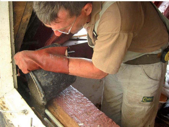
Modern restoration techniques can prevent the need to replace authentic parts.
