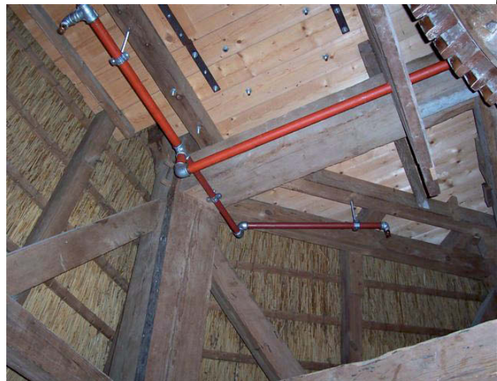
Some mills are equipped with a sprinkler system.
