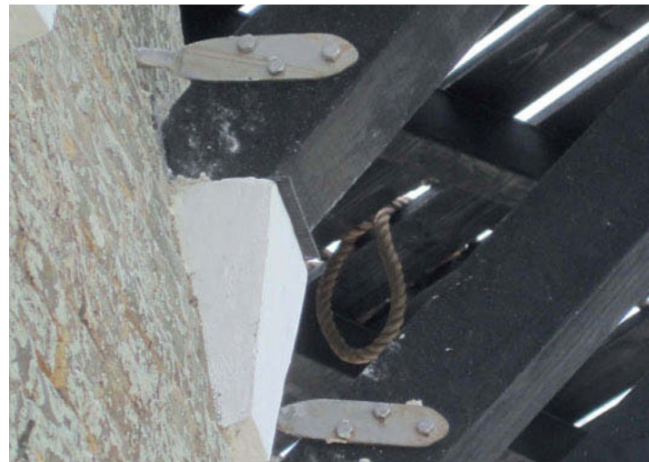
The gallery main shore cramps made of stainless steel.
