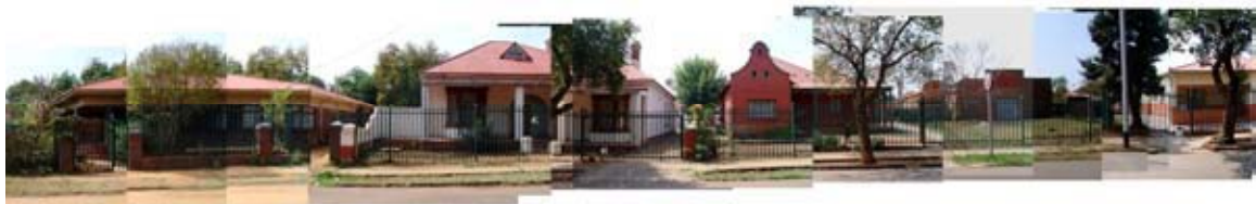
Panoramic view on De Waal Street
